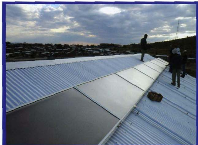
One row of collectors installed
