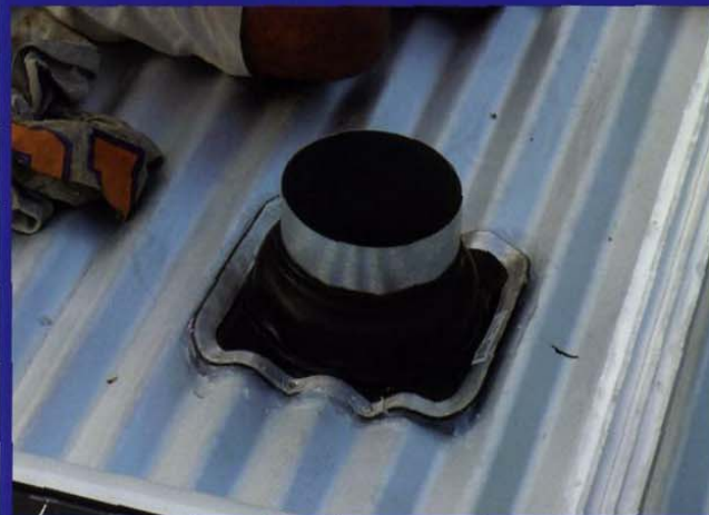
Dektite roof seal for ducting tube
